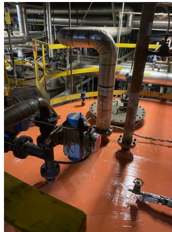
Tank top after one coat of Belzona 5871.
