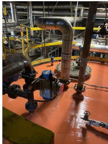
Tank top after one coat of Belzona 5871.
