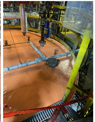
Finished application of Belzona 5871
