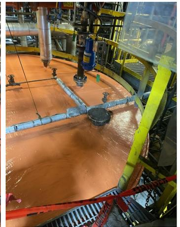
Finished application of Belzona 5871
