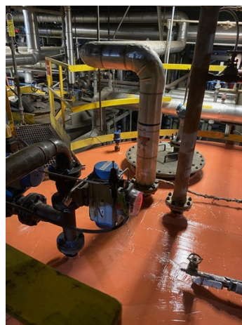
Tank top after one coat of Belzona 5871.
