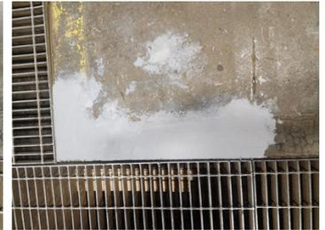
Belzona 4111 application completed.
