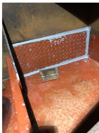
Plate applied to the corroded area
