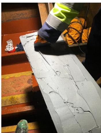
Belzona 1111 applied to plate
