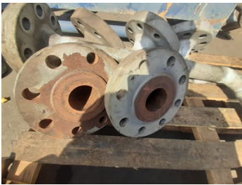
Initial condition of flanges
