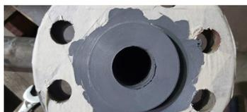
Flange faces rebuilt and restored using forming technique
