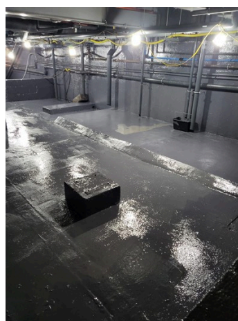
Final coat of Belzona 4311
