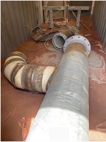
The carbon steel pipes that needed to be coated
