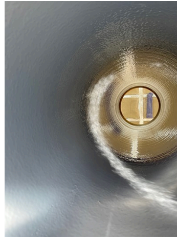
Internal coating of Belzona 5821 on pipe
