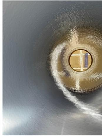
Internal coating of Belzona 5821 on pipe
