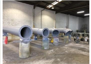
Two coats of Belzona 5821 applied onto external pipes
