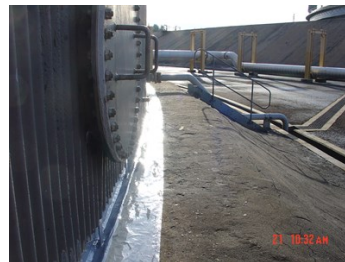
Belzona 3131 applied
