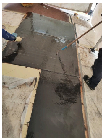
Utilisation of a roller between each layer to remove bubbles and consolidate.
