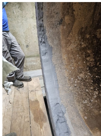
Rebuilding the damage using Belzona 1111.
