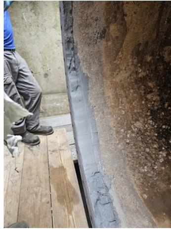
Rebuilding the damage using Belzona 1111.
