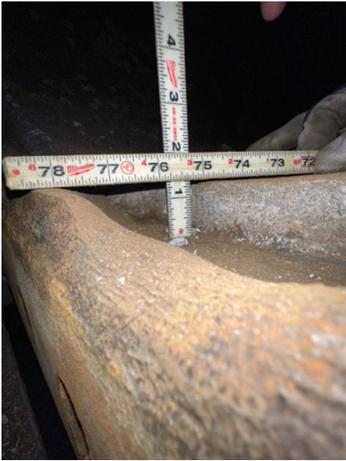
Showcasing and measuring the damage caused by the corrosion.
