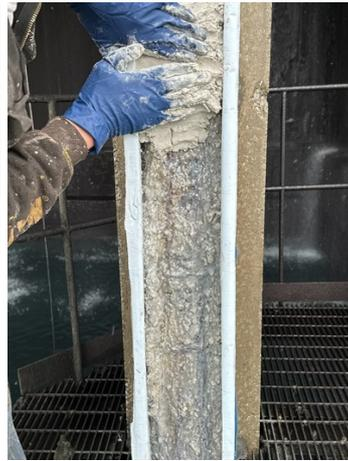
Application of Belzona 4141 for repair
