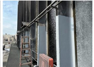
Application of Belzona 5811 for protection
