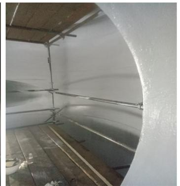
Applying 2 coats of Belzona 1391T
