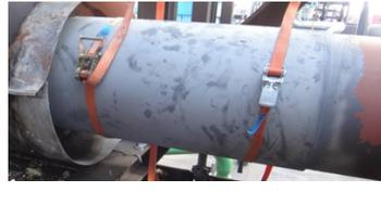
Plate bonded on with Belzona 1511
