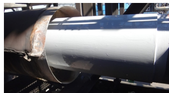
Complete application overcoated with Belzona 5892
