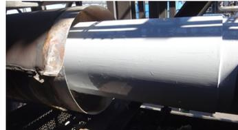
Complete application overcoated with Belzona 5892
