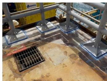
Bonding the small plates with Belzona 7311.
