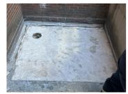
Old Coating was removed and floor was taken to bare concrete by a diamond grinder.
