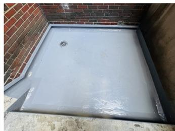
Belzona 3121 with Reinforcement cloth to the seams
