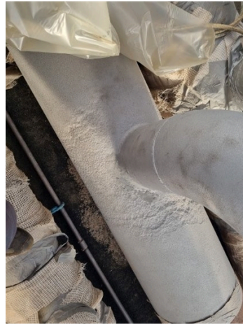
Blasted pipe, ready for superwrap
