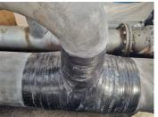
Damadeg pipe Damaged pipe Blasted pipe, ready for Superwrap installed superwrap
