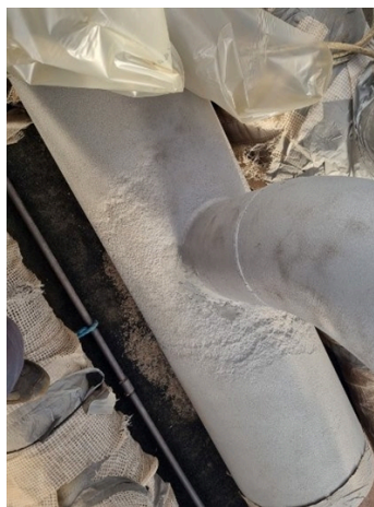
Blasted pipe, ready for superwrap
