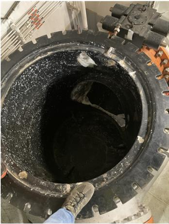
Flaking and damaged lining
