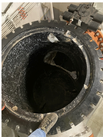
Flaking and damaged lining
