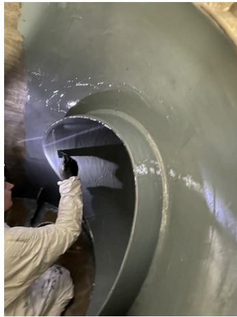
First layer of Belzona 1321 Ceramic S-Metal in progress
