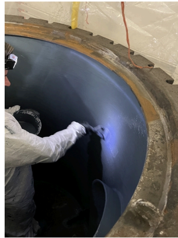
Second layer of Belzona 1321 Ceramic S-Metal in progress
