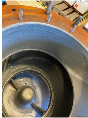
Rebuilding in progress
