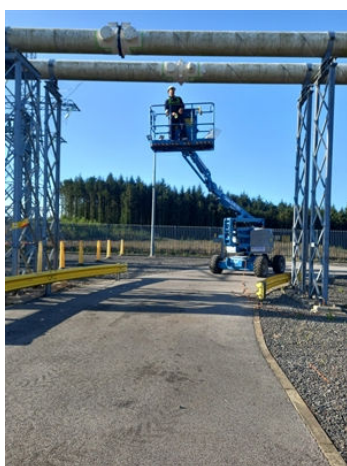
Access, cleaning & roughening of existing system
