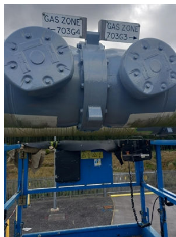
Belzona 5111 1st coat
