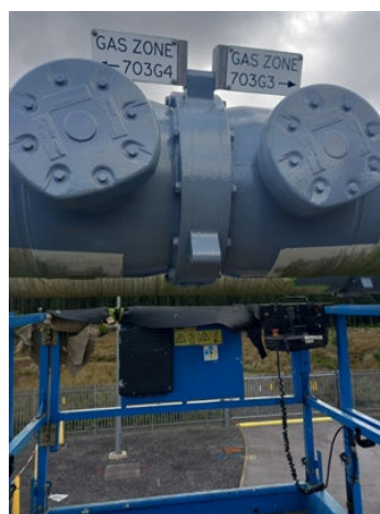
Belzona 5111 1st coat
