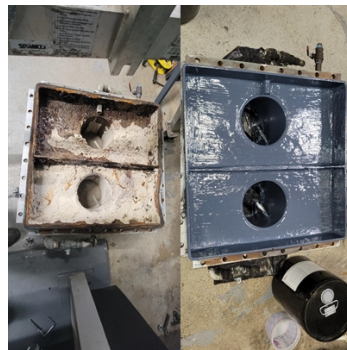
Before and after Belzona application
