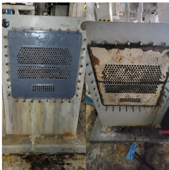
Before and after Belzona application
