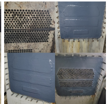
Before and after Belzona application
