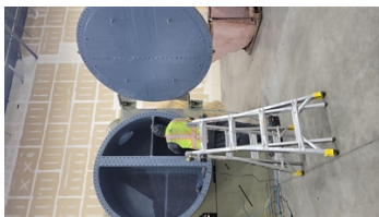
Application of Belzona 1321
