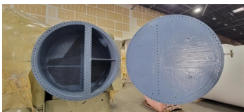
Application of Belzona 1321
