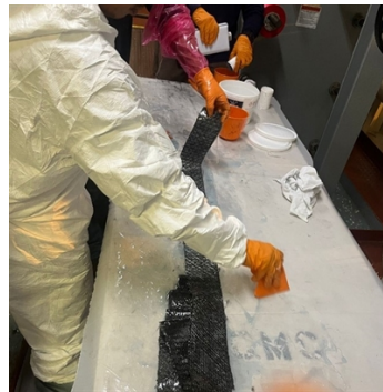
Mixing and and wetting of the Superwrap 2 inside the ship
