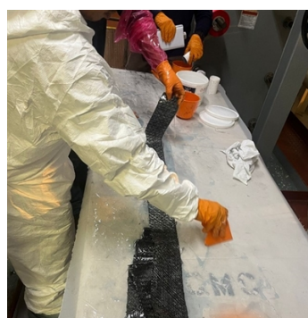
Mixing and wetting of the Superwrap 2 inside the ship
