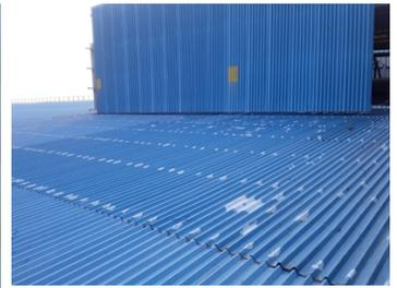
Tin roof required a repair on anchor bolts and joints to prevent water ingress
