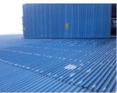
Tin roof required a repair on anchor bolts and joints to prevent water ingress
