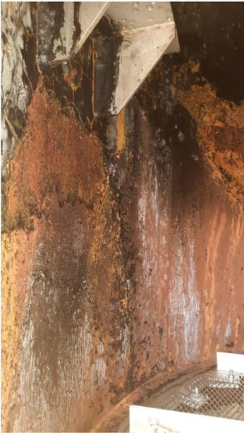
Traces of severe corrosion from under the rubber lining
