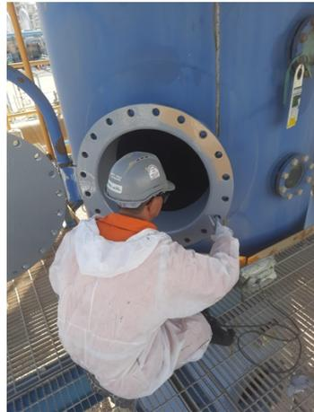
Coating application in progress to the manway and flange
