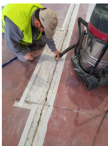
Cleaning after the preparation to remove dust and small debris
