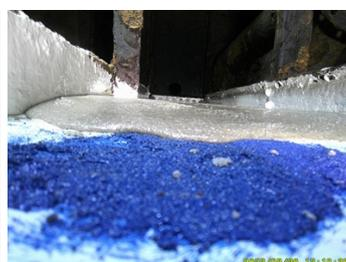
Belzona 4151-silica mixture was poured over Belzona 5831LT and 1818
