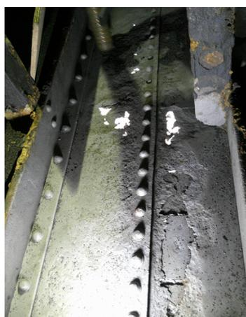
Extensive damage revealed at the tank bottom after blasting
