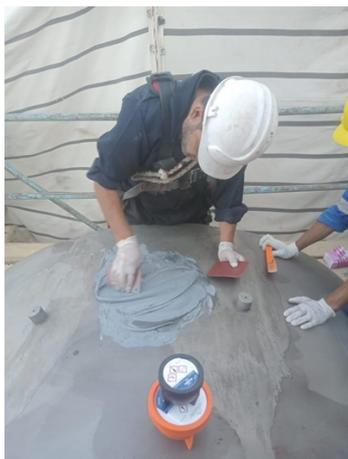
Applying Belzona 1111
