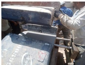
Aligning the tiles to be used as a mould
