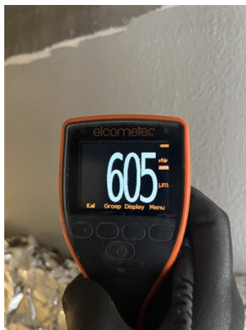
Completed application with coating thickness being checked.
