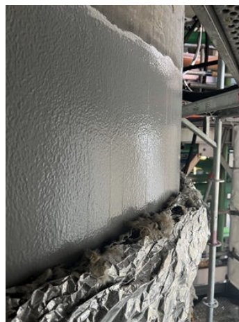
Completed coating with insulation reinstalled.
