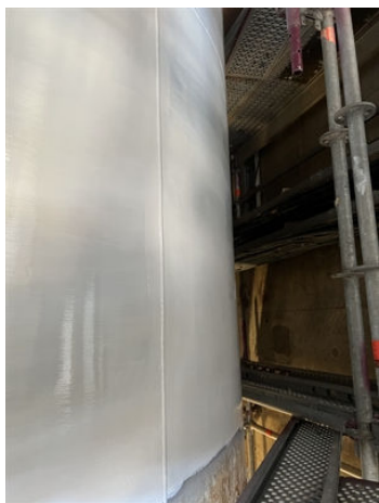
First coat of Belzona 5892 in white.
