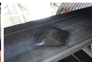
Example of a completed repair
