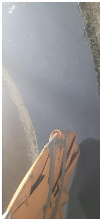
With first coat of Belzona 1321
