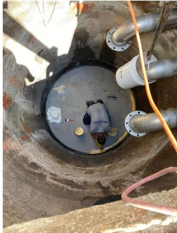
Applying Belzona 4111 (Magma Quartz) and Belzona 5821
