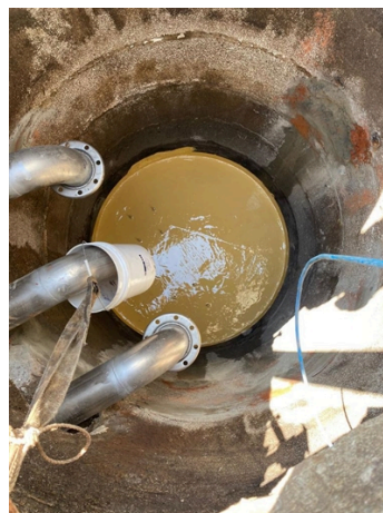
Applying Belzona 4111 (Magma Quartz) and Belzona 5821
