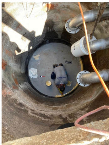
Applying Belzona 4111 (Magma Quartz) and Belzona 5821
