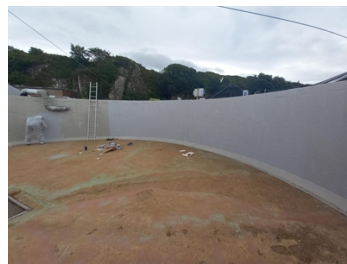
Belzona 5811DW2 application in progress
