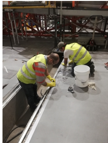
Applying Belzona 4111 (Magma-Quartz)
