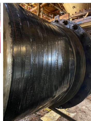
Completed temporary solution for cracked and worn bellow
