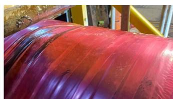
Consolidation film wrapped around SuperWrap II application to ensure adhesion
