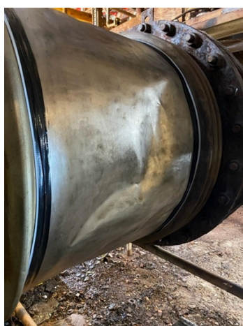
Crack in the bellows terminated and filled with Belzona 1511
