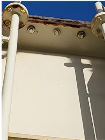
Typical corrosion at the main flange
