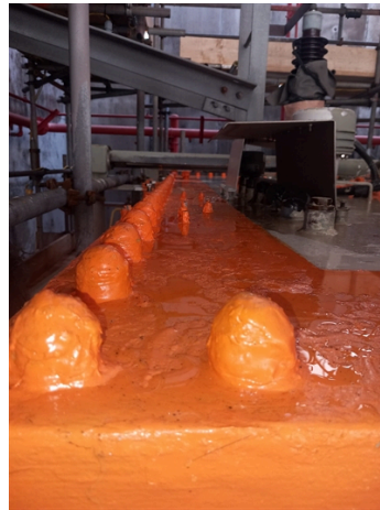
Close up of Belzona 3412 seal on the flange
