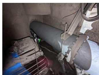
Resurfaced with Belzona 1121
