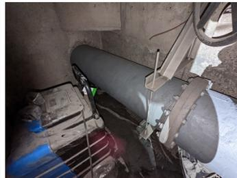
Resurfaced with Belzona 1121
