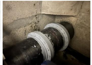
Application completed with SWII reinforcement and coated flanges
