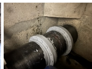
Application completed with SWII reinforcement and coated flanges
