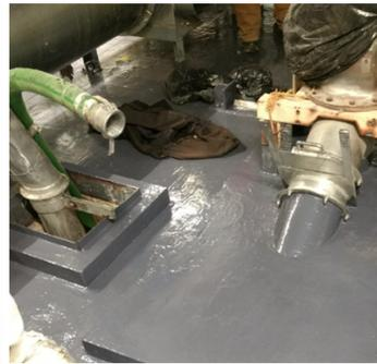
Second coat of Belzona 4311 around floor step up's and piping equipment through floor.
