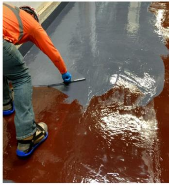
Applying second coat of Belzona 4311
