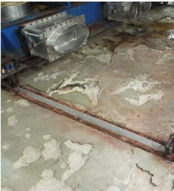
Floor damage caused by Succinic Acid
