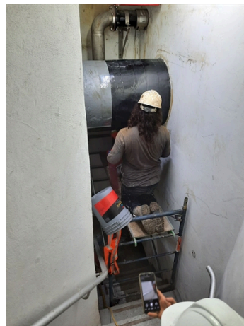
1st layer of Belzona SWII
