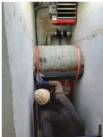
Plate bonding over the most critical area
