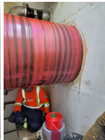
Complete repair after consolidating with the release film to be later removed
