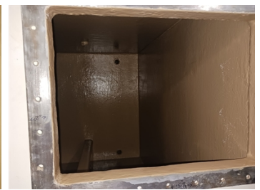
Black Tank After application of two coats of Belzona 5811.
