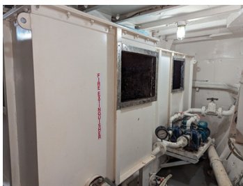
Tanks before surface preparation.
