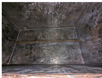
After surface preparation.
