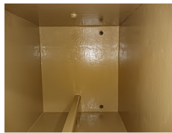
Gray Tank After application of two coats of Belzona 5811.
