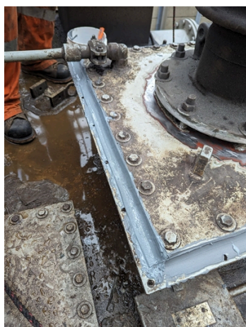
Leaks stemmed and sealed with Belzona 1161
