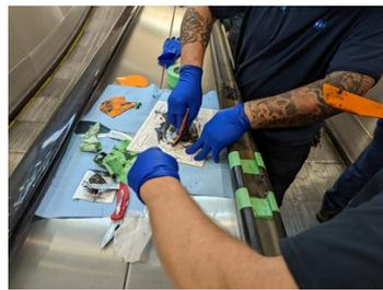
Mixing of Belzona 2311
