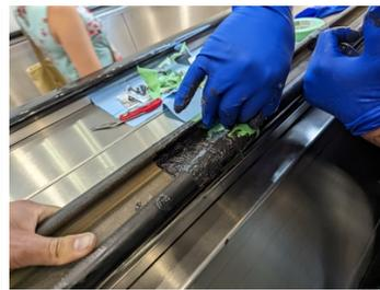
Removing masking tape after applying 2311
