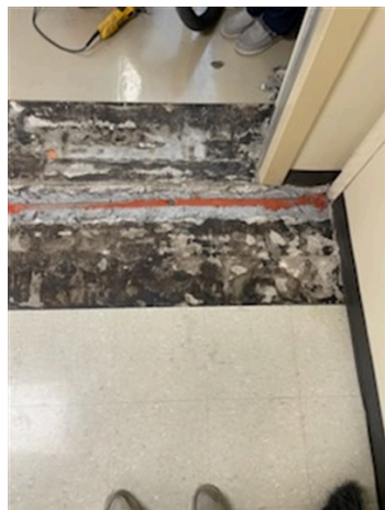
Removing existing expansion joint
