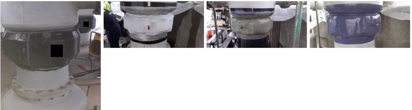
Previous repair was leaking SF6 gas around the edges of the bond area.
