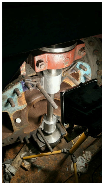
Belzona 1121 applied with formers in place
