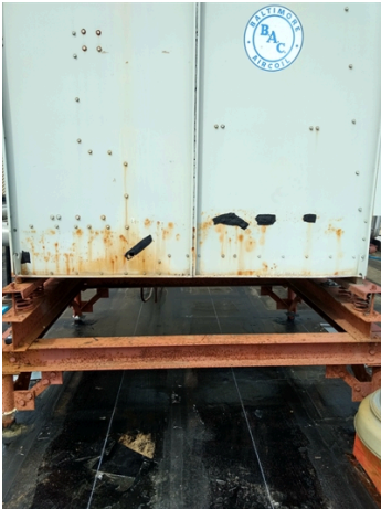
Damaged cooling tower
