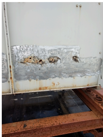
Surface preparation with a grinder over the affected area
