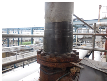
Completed repair with Belzona 1981 SuperWrap 2 installed
