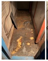
Surface preparation to reveal holes in pan and ready for cold plate bonding.
