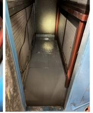
First coat of Belzona 5831LT White applied. Second coat of Belzona 5831LT Grey applied.
