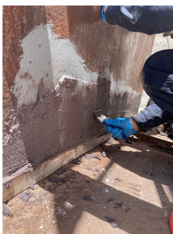
Area being prepared for application of Belzona 1212 and plate bond with Belzona 1812.
