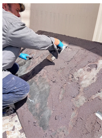
Belzona 1812 being applied to prepared plate to get ready to bond it to the chute.
