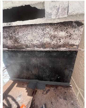
Job complete. Belzona 1212 and reinforcement cloth used to repair holes then a plate was boned with Belzona 1812 for abrasion protection.
