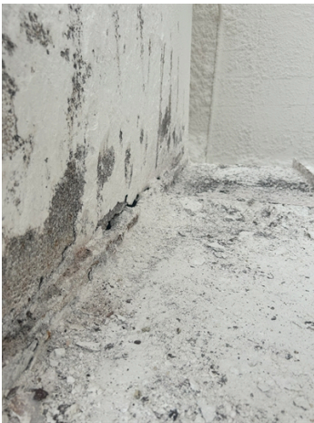
Area before being cleaned and prepared for work.
