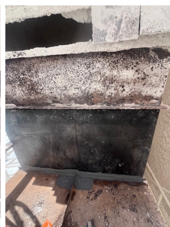
Job complete. Belzona 1212 and reinforcement cloth used to repair holes then a plate was boned with Belzona 1812 for abrasion protection.
