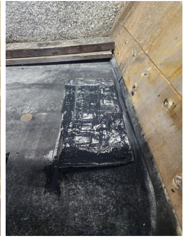
Belzona 2211 application completed.
