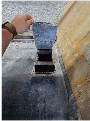
Lifting the torn flap of the conveyor belt to show the extent of the damage.
