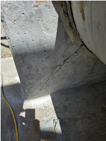
Power plant water cooling pipe pedestal and crack
