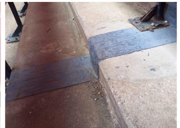
The original issue, with all loose and friable removed, ready for repairs to be made and a 30mm gap to be created
